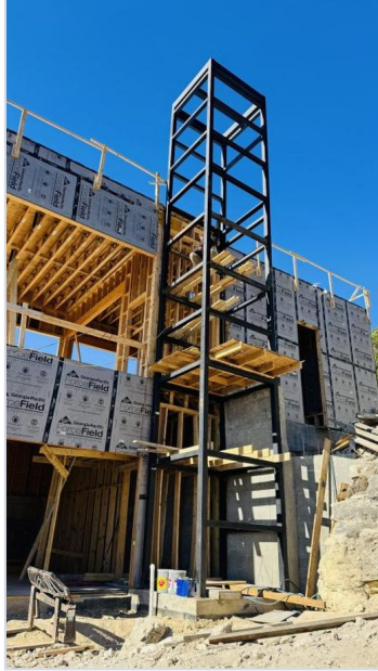
Welded steel tower structure
