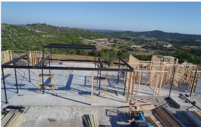
Structural steel framing — custom residential build
